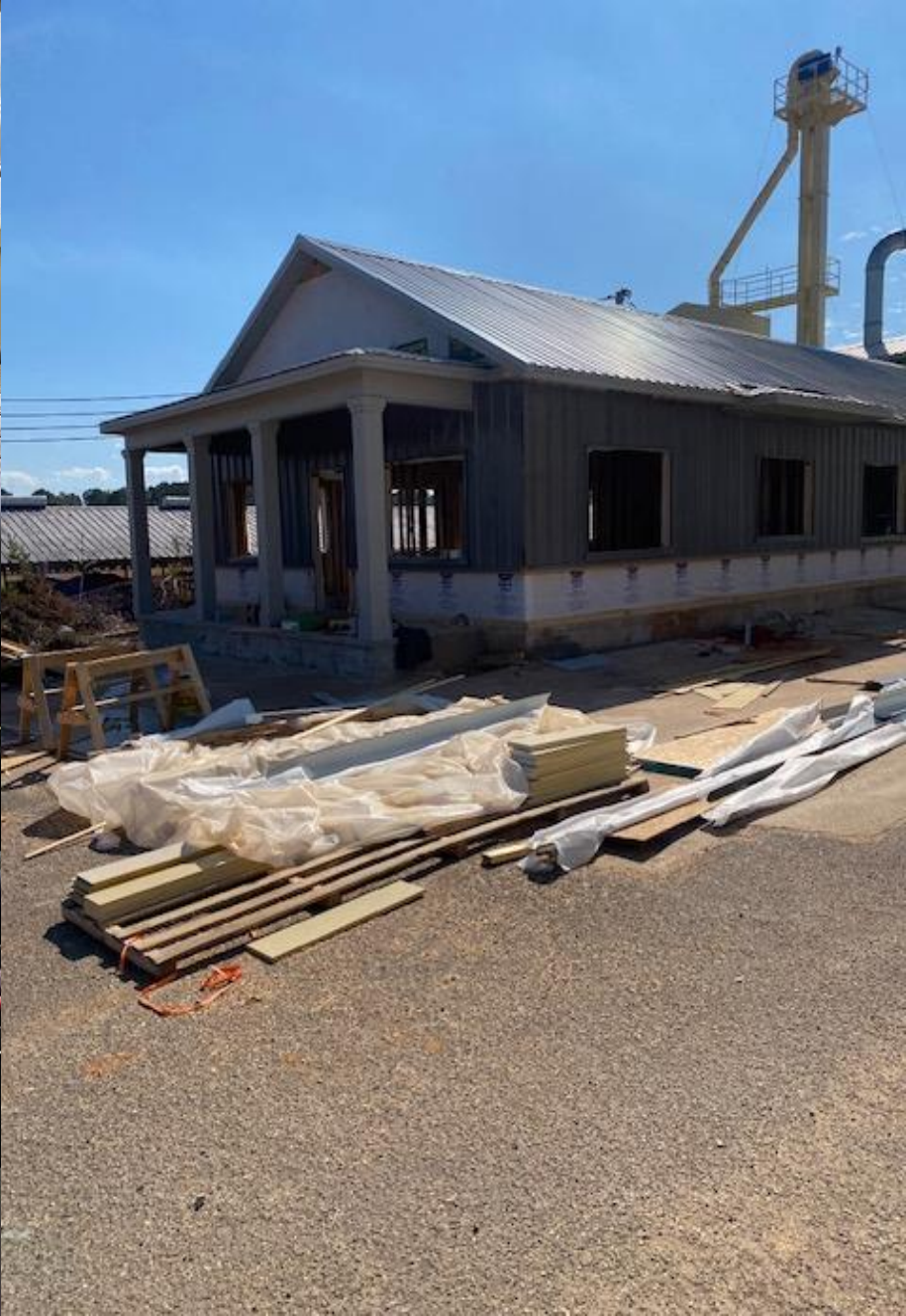
Plains Office Remodel 2024
